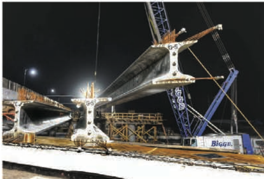
Laying the girders for Highway 101
