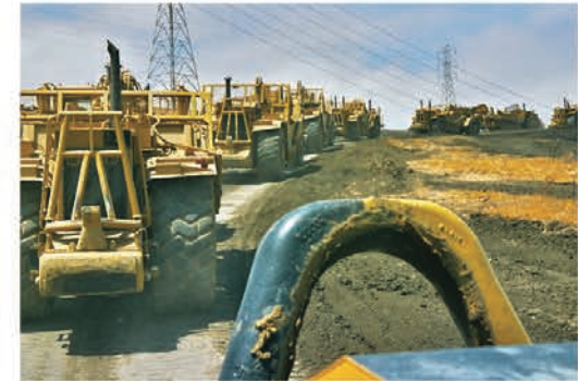
Ghilotti scraper fleet moving millions of yards of dirt at San Marcos in Pittsburg, CA
